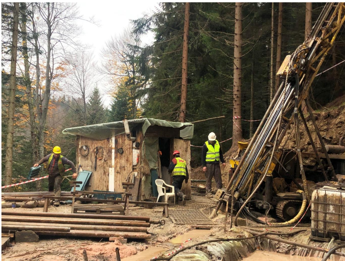
Photo 5.11.2: Drilling Rig in Rupice Forested Area
